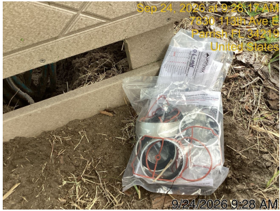
Old parts removed Pond 11
