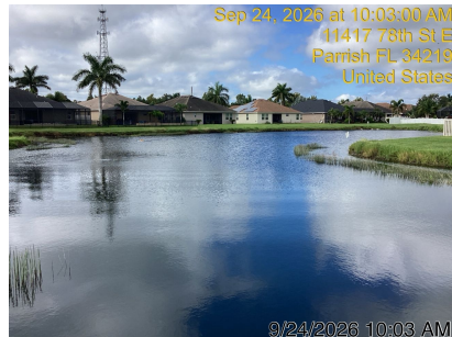
Pond 10 Both diffusers working
