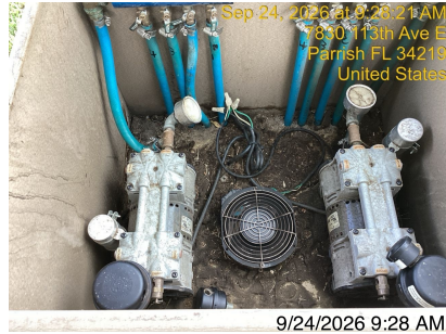
Both compressors rebuilt Pond 11
